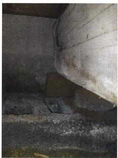
Photograph (17): Poorly supported earing condition at center girder (north end).
