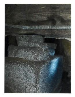
Photograph (16): Poorly supported bearing condition at center girder (mid-span).
