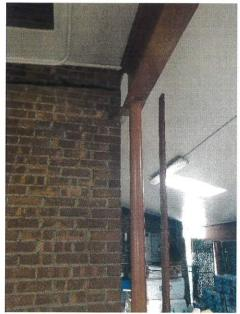
Photograph (9): Damaged brick masonry at canopy steel.
