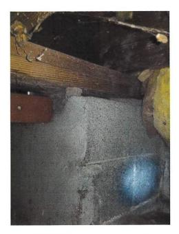
Photograph (18): Poorly supported sill plate. Displaced insulation. Representative conditions.
