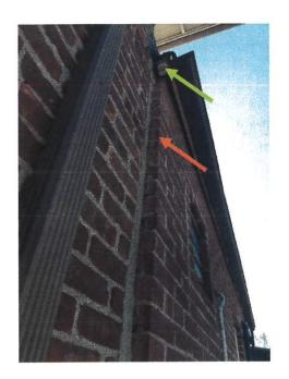
Photograph (7): Reported displacement at kitchen addition (red arrow). Deteriorated wood curb / blocking (green arrow).
