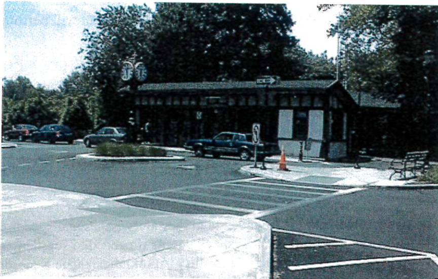
Curb bumpouts installed in Scarsdale.
