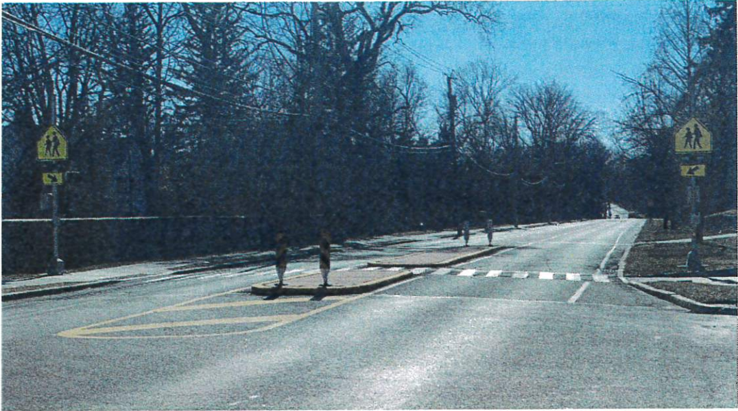
Crosswalk with RRFB's on conjunction with a Road Diet installed in Rye.
