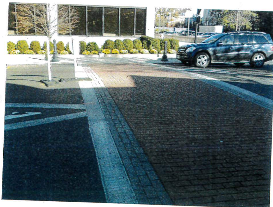
Raised Crosswalk installed in Greenwich.
