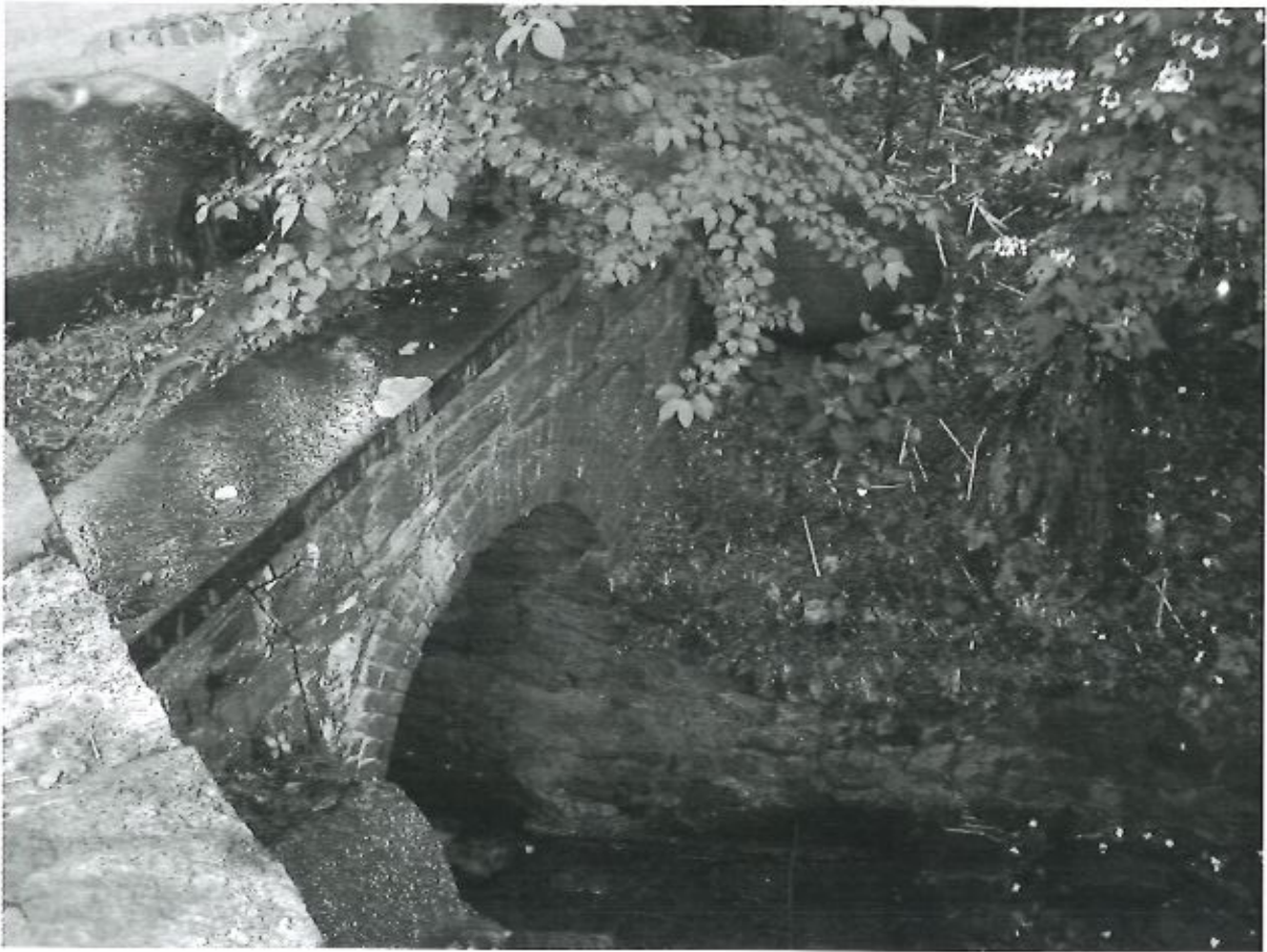
Lower culvert stone and brick inlet.
