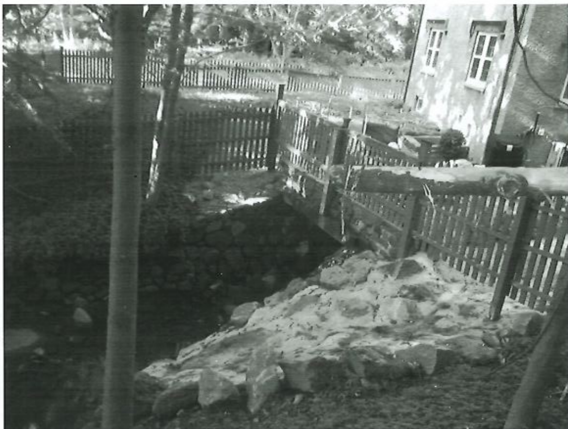
Lower culvert outlet (post restoration from Tropical Storm Ida)
