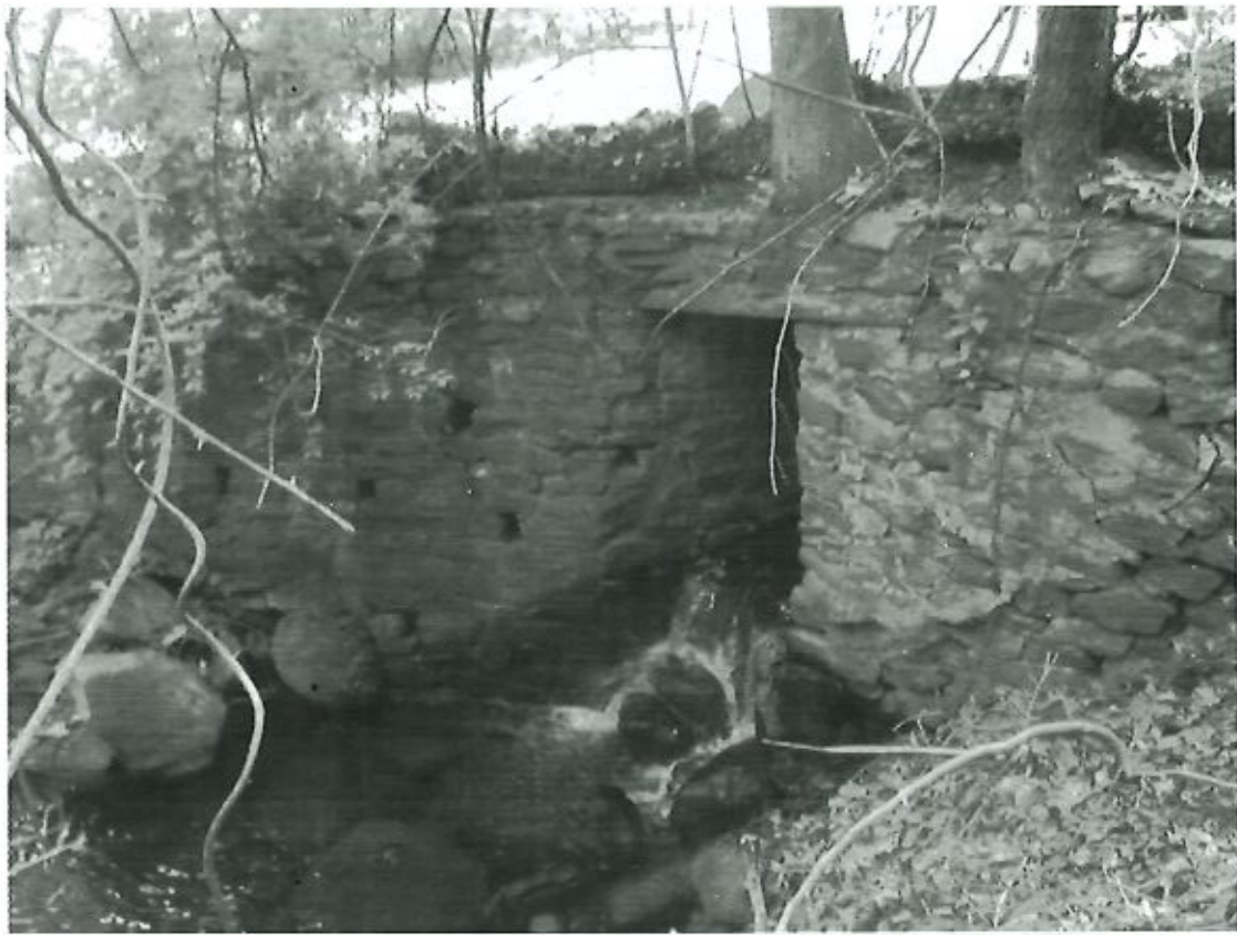
Upper culvert outlet.
