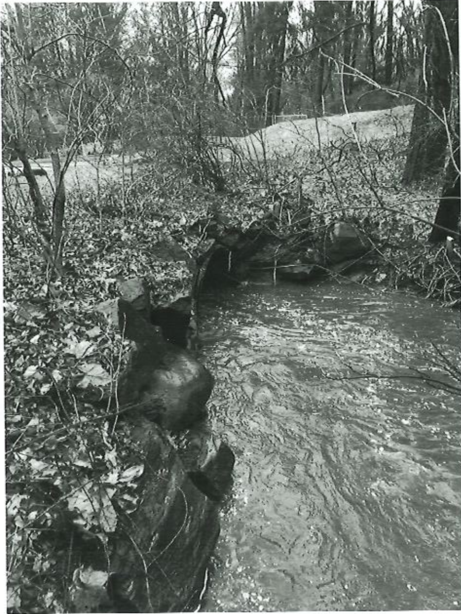
Upper culvert inlet.
