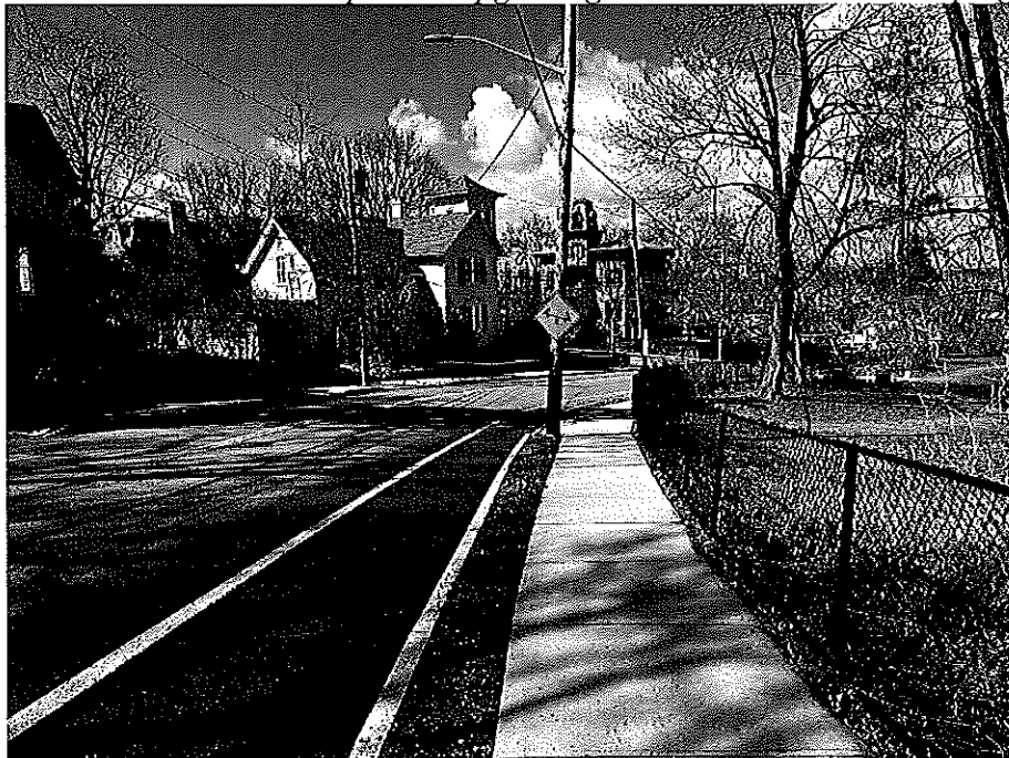
Looking right from potential crosswalk location on Neperan Road opposite Altamont Avenue. Note that the photo was taken in the winter and the area will have more vegetation during the warmer months which will further hinder sight distance.
