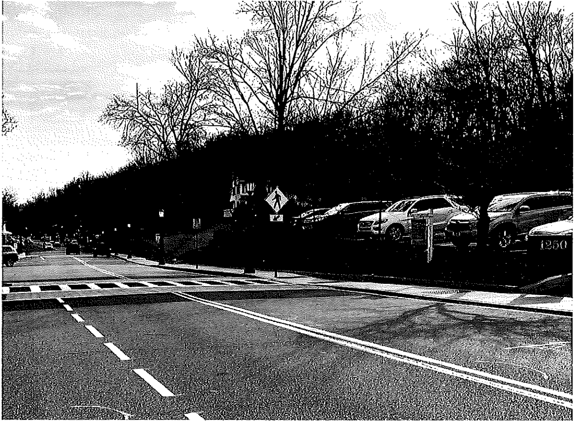
Example of a slightly raised high-visibility crosswalk
