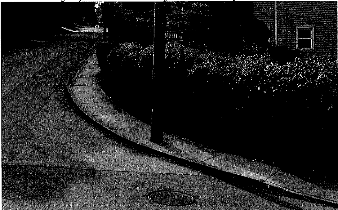
Utility pole in middle of sidewalk.
