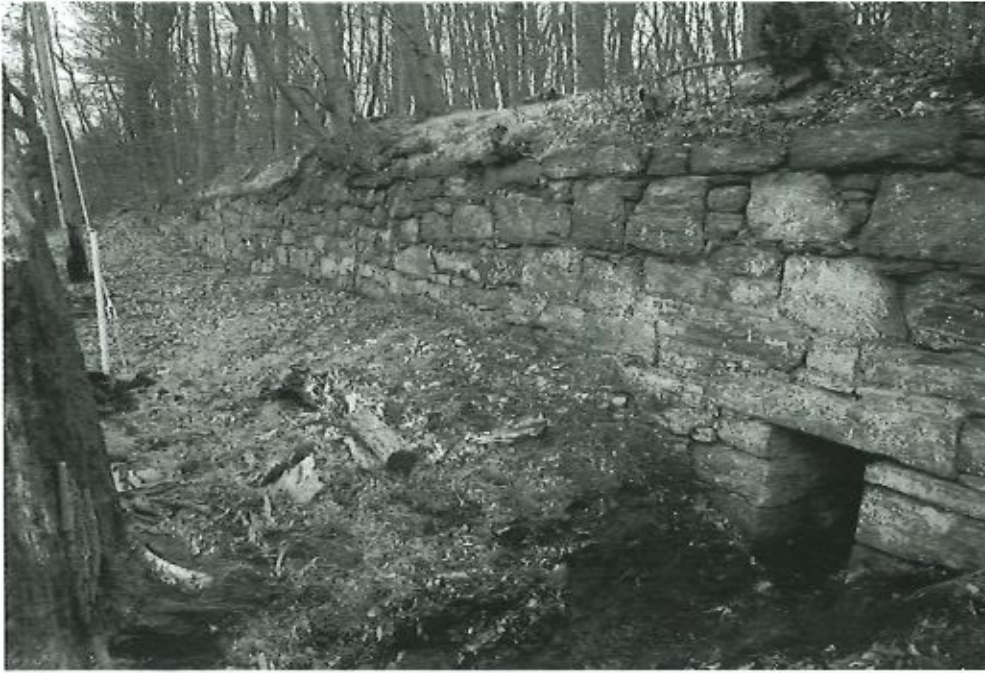
Photo 11 Dam ID# 214-0271 Tarrytown Waterworks Dam 02/07/2023 Auxiliary Spillway Outlet Looking upstream
