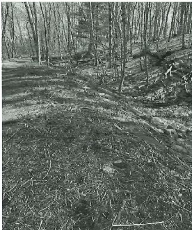
Photo 3 Dam ID# 214-0271 Tarrytown Waterworks Dam 03/09/2023 Auxiliary Spillway Channel Looking downstream
