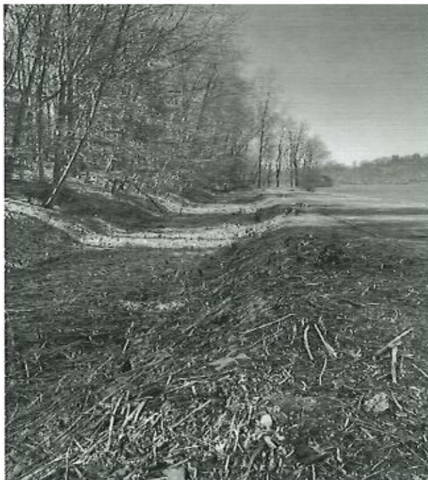
Photo 4 Dam ID# 214-0271 Tarrytown Waterworks Dam 03/09/2023 Auxiliary Spillway Channel Looking upstream
