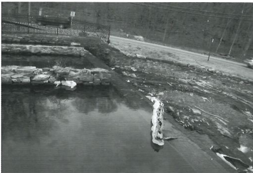
Photo 5 Dam ID# 214-0271 Tarrytown Waterworks Dam 02/07/2023 Service Spillway
