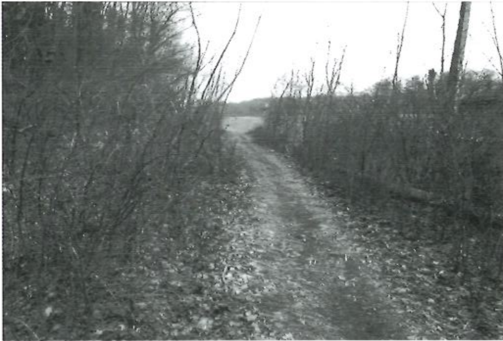
Photo 9 Dam ID# 214-0271 Tarrytown Waterworks Dam 02/07/2023 Auxiliary Spillway Channel Looking upstream
