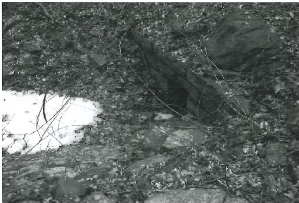
Photo 10 Dam ID# 214-0271 Tarrytown Waterworks Dam 02/07/2023 Auxiliary Spillway Outlet Looking downstream
