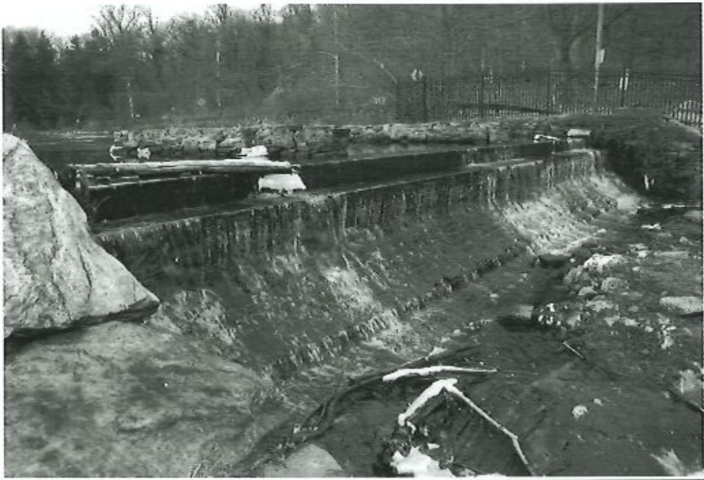
Photo 4 Dam ID# 214-0271 Tarrytown Waterworks Dam 02/07/2023 Service Spillway
