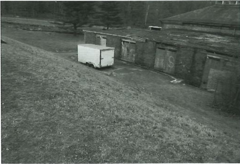
Photo 3 Dam ID# 214-0271 Tarrytown Waterworks Dam 02/07/2023 Downstream Embankment
