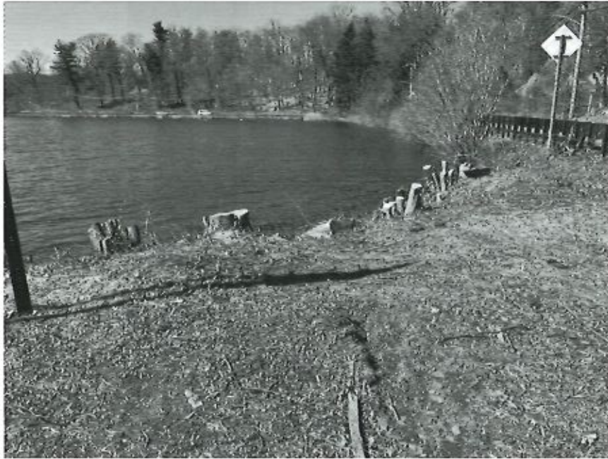
Photo 5 Dam ID# 214-0271 Tarrytown Waterworks Dam 03/07/2023 Service Spillway Looking upstream
