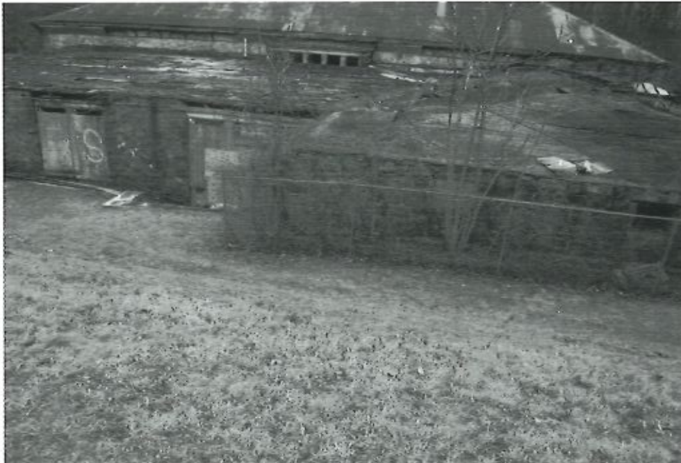
Photo 2 Dam ID# 214-0271 Tarrytown Waterworks Dam 02/07/2023 Downstream Embankment
