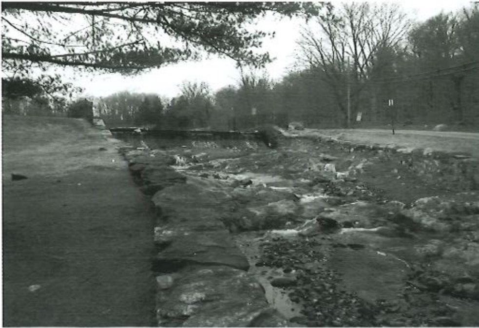
Photo 7 Dam ID# 214-0271 Tarrytown Waterworks Dam 02/07/2023 Service Spillway Channel
