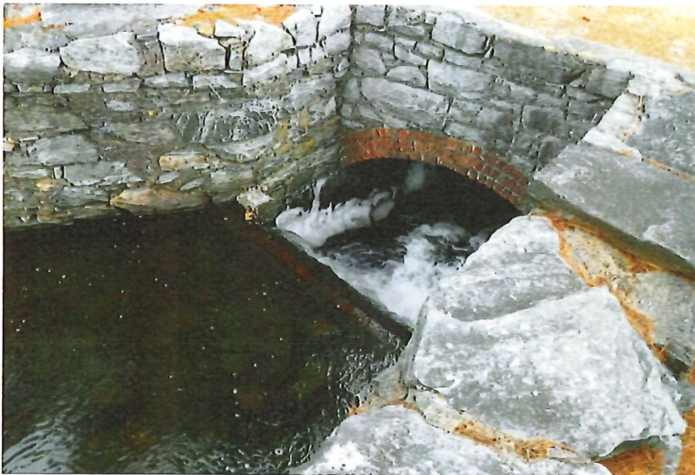
Photo 6 Dam ID# 214-0271 Tarrytown Waterworks Dam 02/07/2023 Culvert Downstream of Service Spillway
