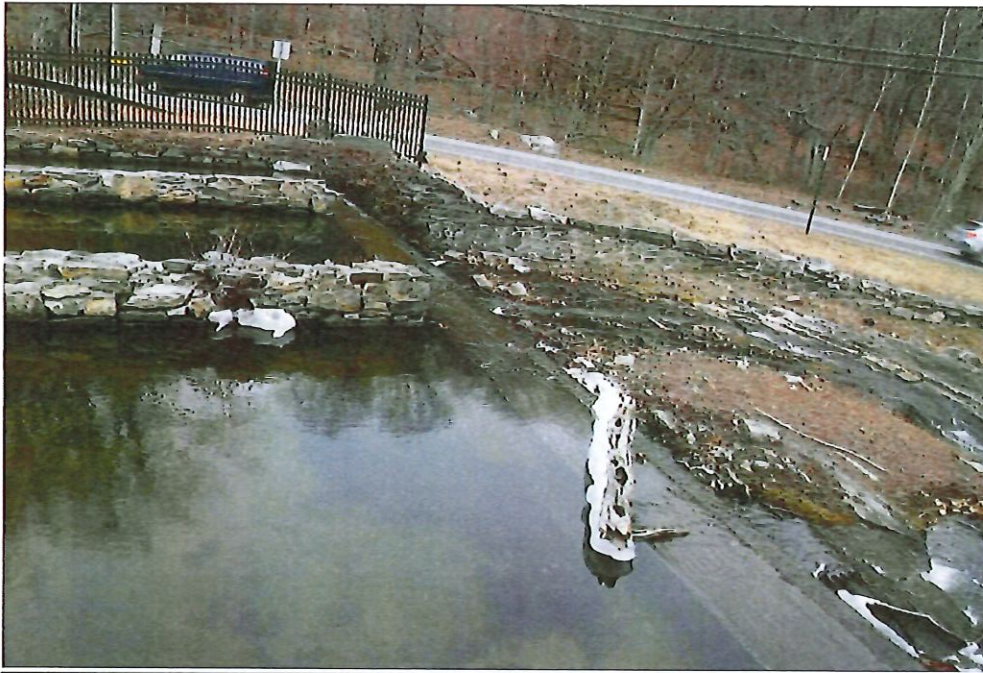
Photo 5 Dam ID# 214-0271 Tarrytown Waterworks Dam 02/07/2023 Service Spillway
