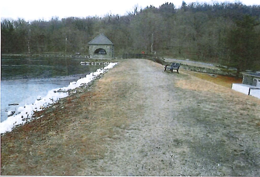
Photo 1 Dam ID# 214-0271 Tarrytown Waterworks Dam 02/07/2023 Upstream Embankment and Dam Crest
