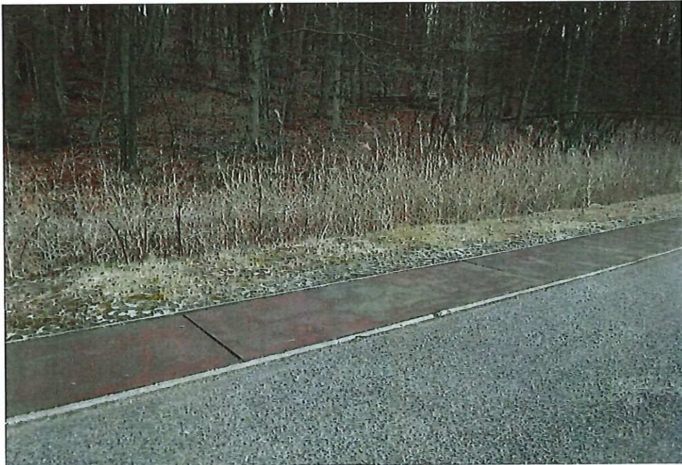
Photo 8 Dam ID# 214-0271 Tarrytown Waterworks Dam 02/07/2023 Auxiliary Spillway Entrance
