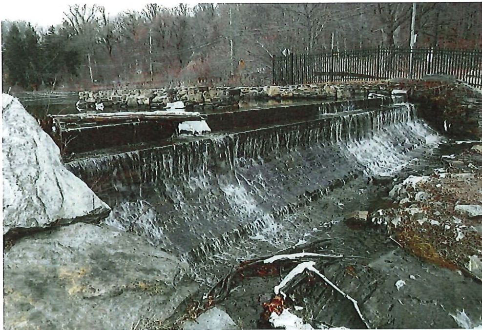
Photo 4 Dam ID# 214-0271 Tarrytown Waterworks Dam 02/07/2023 Service Spillway
