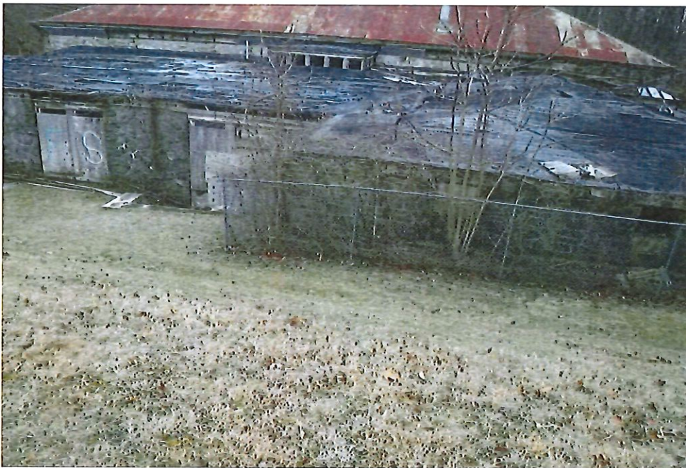
Photo 2 Dam ID# 214-0271 Tarrytown Waterworks Dam 02/07/2023 Downstream Embankment
