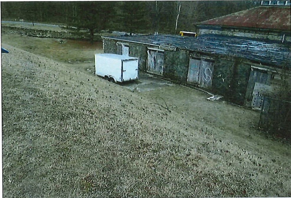
Photo 3 Dam ID# 214-0271 Tarrytown Waterworks Dam 02/07/2023 Downstream Embankment
