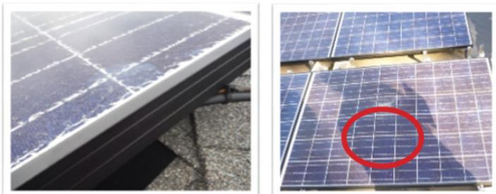
**Photo 5** - Conductors over 30V not guarded, installed in raceway, or otherwise inaccessible: NEC 690.31(A)
