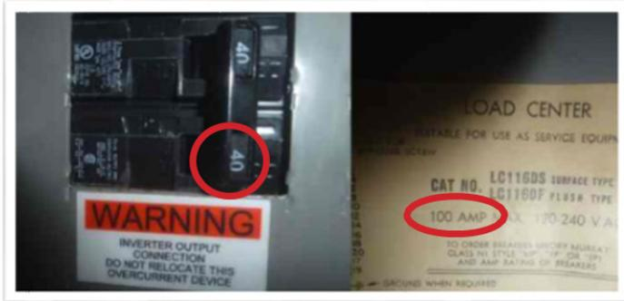
**Photo 2:** Backfed PV breaker not installed at opposite end of buss bar from main breaker: NEC 705.12(B)(3)(b)
