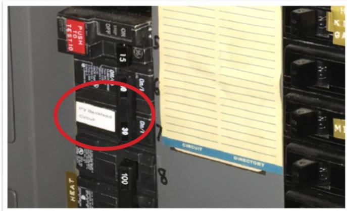
**Photo 3:** Working clearance not maintained: NEC 110.26
