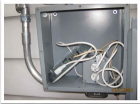
**Photo 10:** DC Conductor in contact with sharp edge: NEC 334.15(B)
