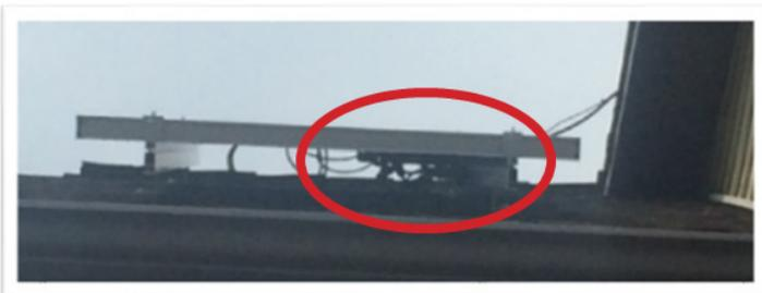
**Photo 9:** Equipment is not rated for location. In this case, a non-GFCI outlet for PV monitoring equipment is located in a wet location: NEC 110.3(B), 210.8(A)(3)
