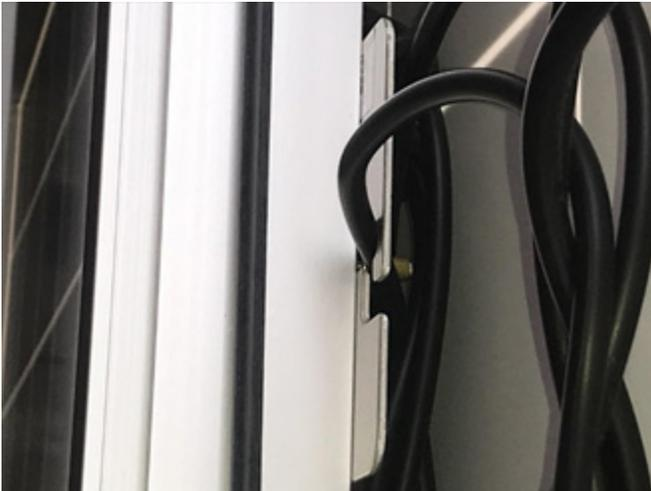
**Photo 11:** AC disconnect/load center manufacturer's label obscured: NEC 110.21
